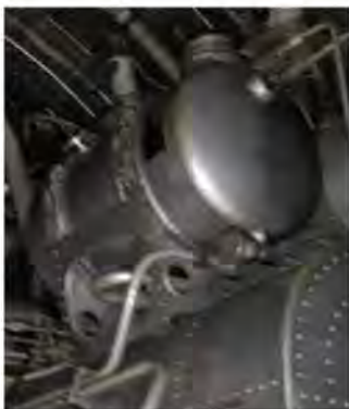
Two 1.5 kg Freon filled fire extinguishing bottles protect each engine
